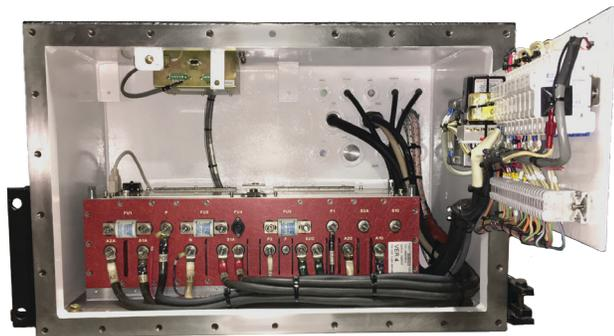
Q750 system mounted in XP box with swinging panel closed
